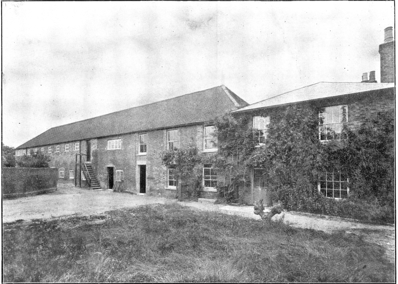
BECK FLAME LAMP LIMITED WORKS AT HAYES, MIDDLESEX.
